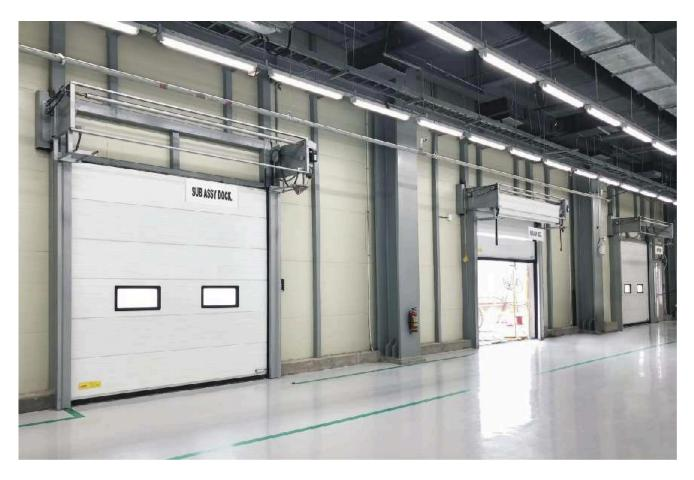
Stacking door is an electrically operated insulated vertically stacking sectional door panels that can be installed in locations where headroom constraints or noise restrictions prevent the use of other conventional industrial doors.
